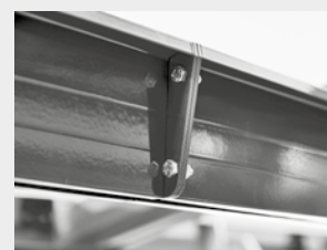
Purlin connection Screws and nuts made of stainless steel
